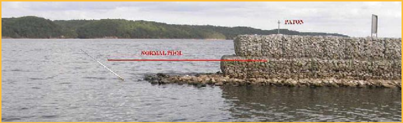
Breakwater at J. P. Coleman State Park Marina with water below normal pool. Good example of value of local knowledge and reason not to take any structure too close aboard. Note position of last PATON on breakwater. Safe water is to the left of the leaning pipe. Photo taken under way from inside harbor by Gary Akin.
